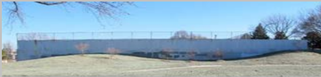
The existing wall in Meldrum Park
