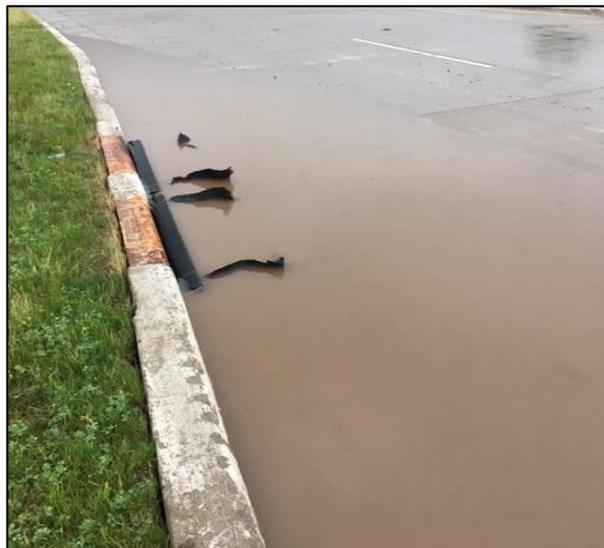
This photo highlights the often overlooked importance of properly functioning inlet protection. The protection used here allowed for a good amount of sediment deposition while continuing to drain the area.
